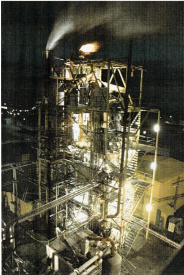
Fig. 11 TPS's CFB gasification and hot gas cleaning pilot plant
